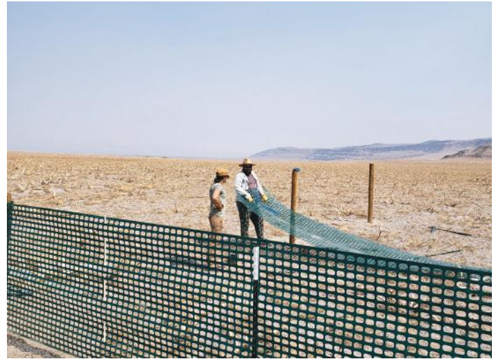
Wind fencing to improve soil stabilization
